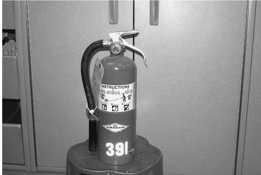
Figure 3-59 Portable extinguishers are marked to indicate what type of fire they should be used on.
