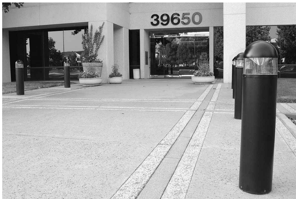
Figure 3-51 Sidewalks, lights, and landscaping can be used for protection.
